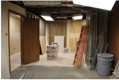
HPWD Office Renovation
